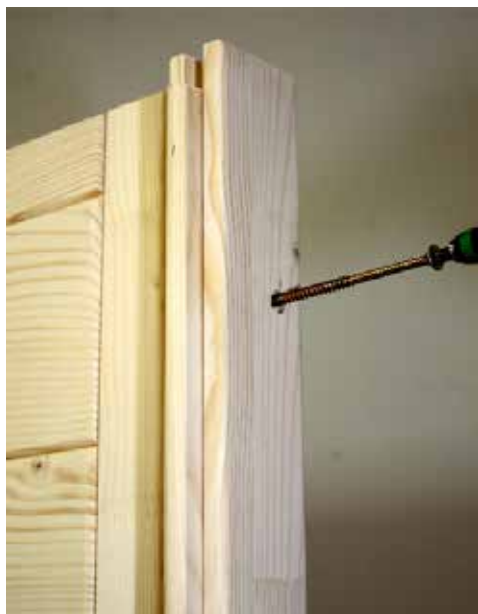
8 screws 6 x 120 mm per corner post
