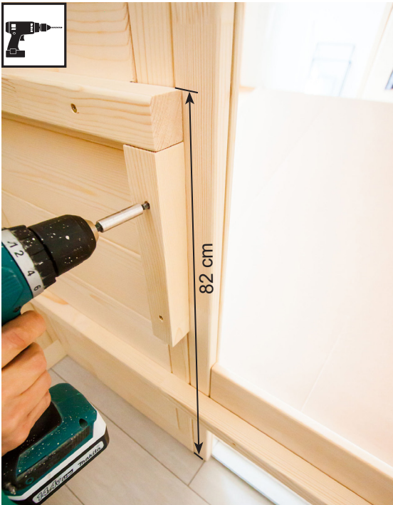
3 screws 5 x 70 mm 2 screws 4 x 60 mm
