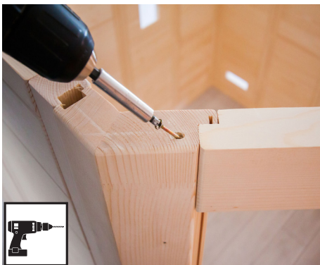
Foret de 3 mm, 1 vis 4 x 70 mm
