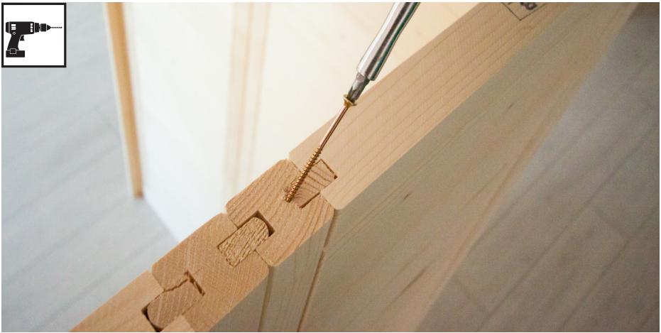
3 mm drill bit, 8 screws 4 x 70 mm
