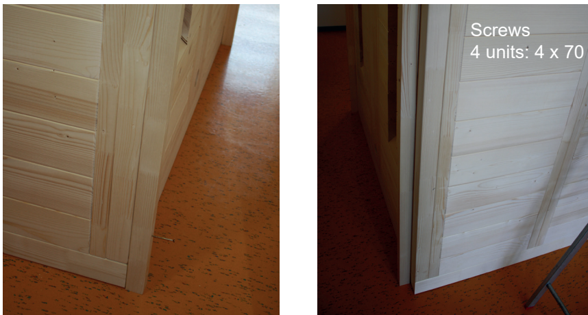
Fig. 46: Installation of the spacer strips of the rear wall
