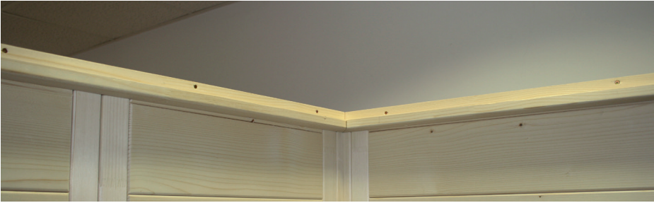
Fig. 16: Installing the roof element in the back with the fan cut-out
