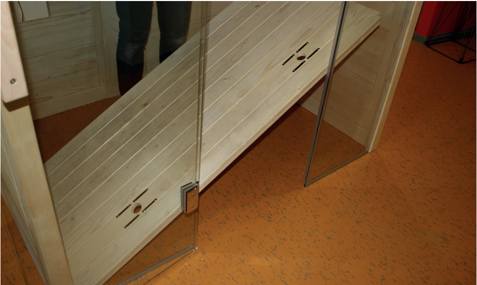
Fig. 26: Put the cabin floor in place
