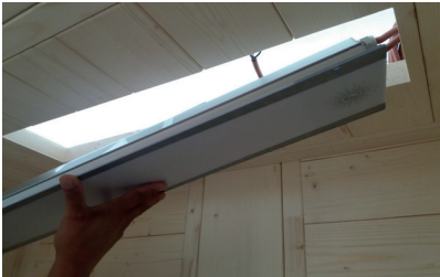
Fig. 44: Installing the colour light
