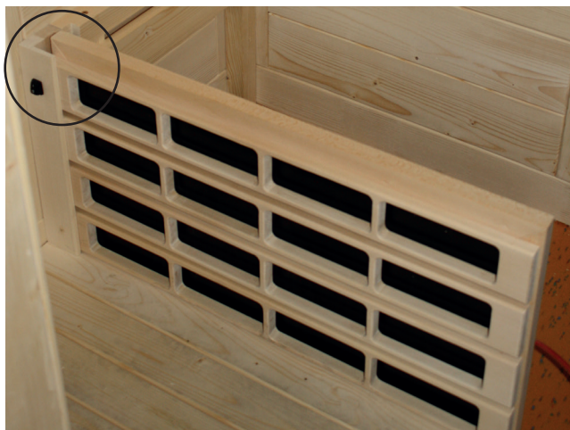
Fig. 32: Installation of the IR thermal plate VitaMy 164
