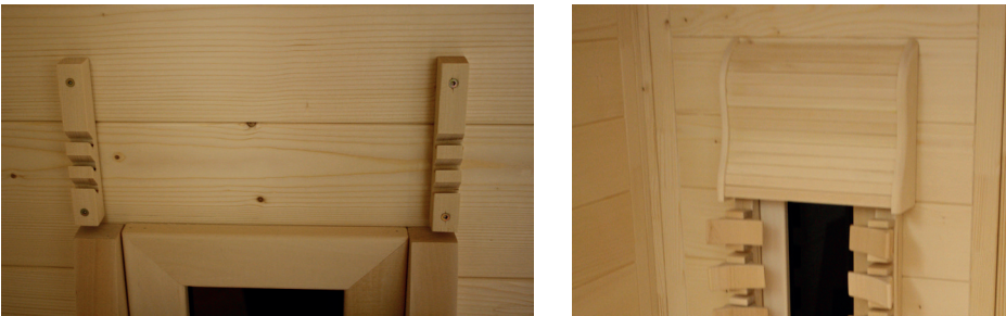
Fig. 47: Installation of the headrests
