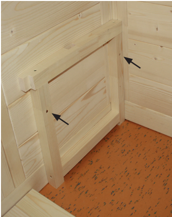
Fig. 30: Installation of the bench cushion
