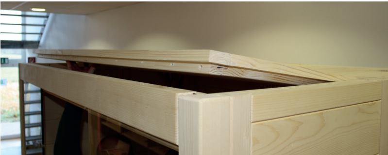
Fig. 17: Installing the roof element in the front
