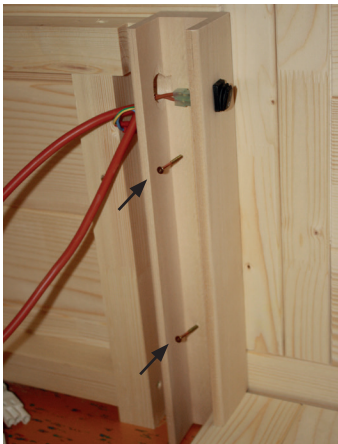
Fig. 31: Installation of the U-strips for the thermal plates
