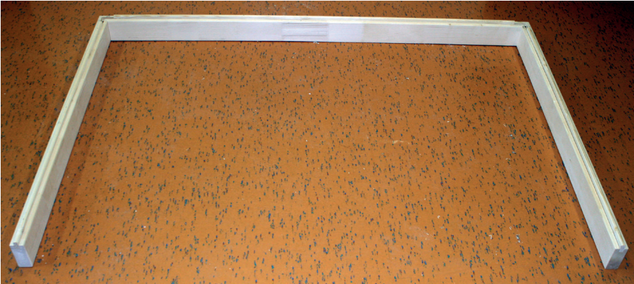
Fig. 1: Placing the three floor frame elements
