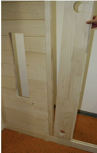
Fig. 6: Install the electrical element in place
