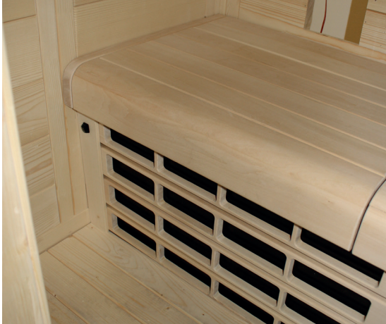
Fig. 35: Inserting the bench
