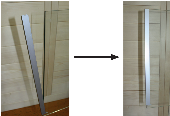
Fig. 10: Attach the U-profiles to the glass plates
