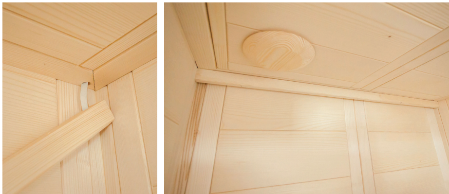
Fig. 41: Attaching the LED strip
