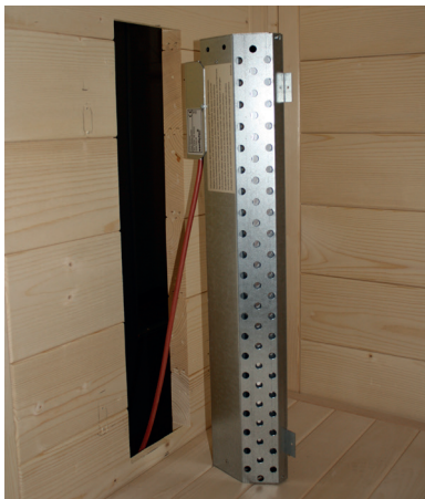
Fig. 36: Install the rear radiator (infrared radiator ECO 350)
