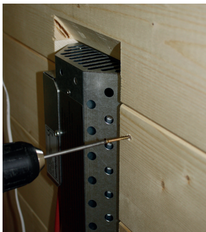
Fig. 37: Installing the read radiator blind
