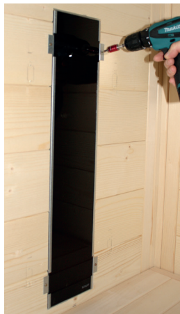
Fig. 36: Install the rear radiator (infrared radiator ECO 350)
